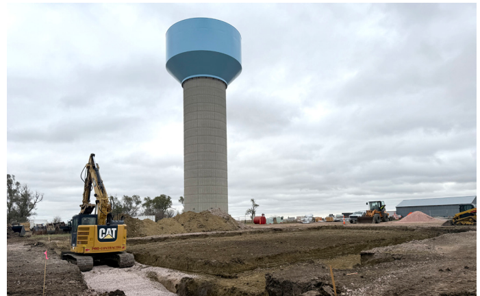
ABOVE: Construction began on the booster station at the Stickney Elevated Tank. (SOURCE: SEH)
