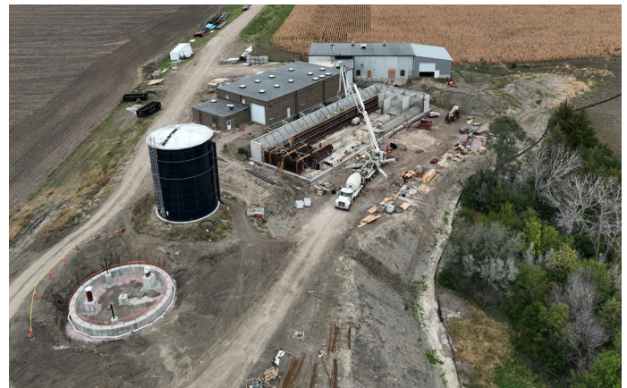
ABOVE: Platte Treatment Plant Progress (SOURCE: TDG)
