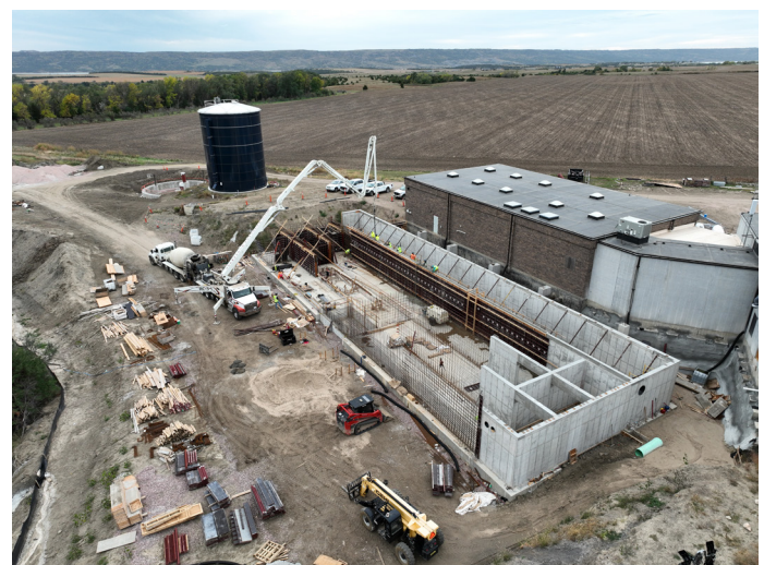
ABOVE: Platte Treatment Plant Progress (SOURCE: TDG)
